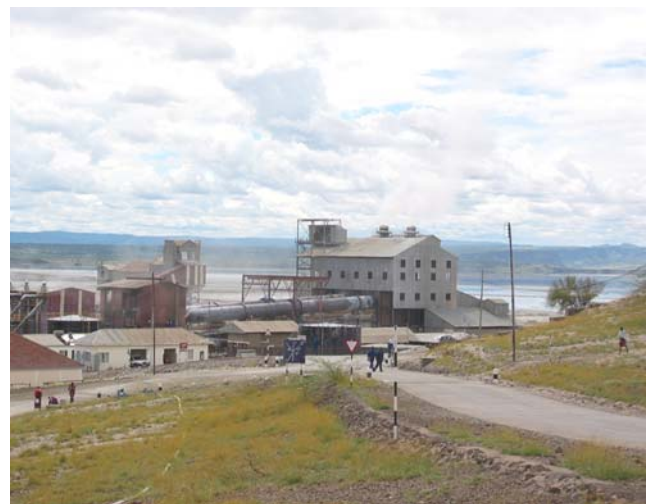
Standard Ash Production Plant
