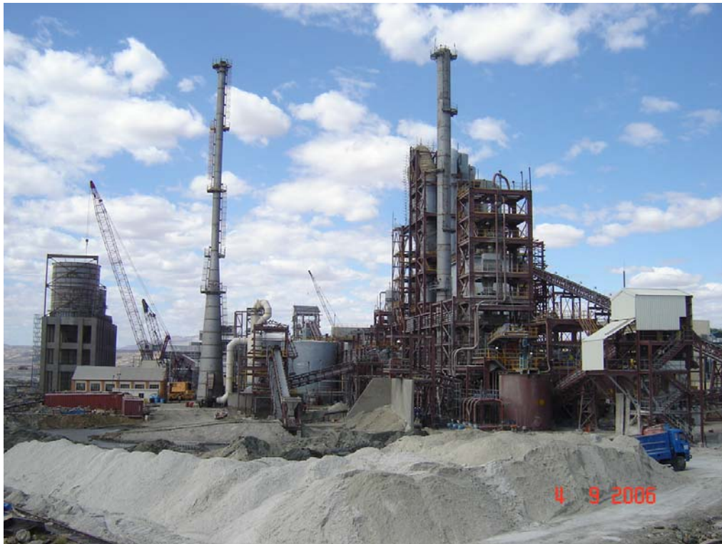
Premium Ash Plant Construction Work in Progress
