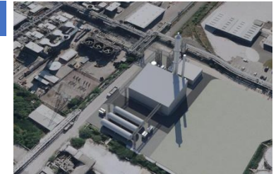
Carbon Capture Utilisation Unit in UK commissioned in Sept 21
